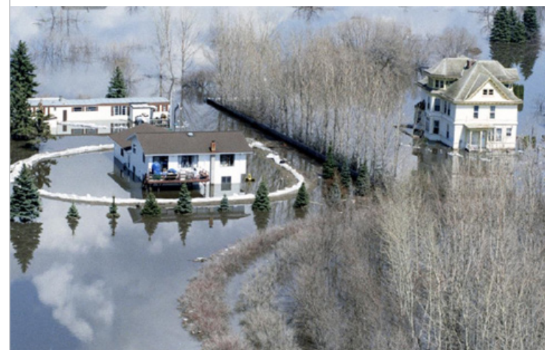
Failed sandbag ring dikes around modern and historic homes after a 1997 major flood in Fargo, North Dakota. Source: Forum file in The Grand Forks Herald February 2020 https://www.grandforksherald.com/news/weather/4929282-Should-you-buy-flood-insurance-this-year
