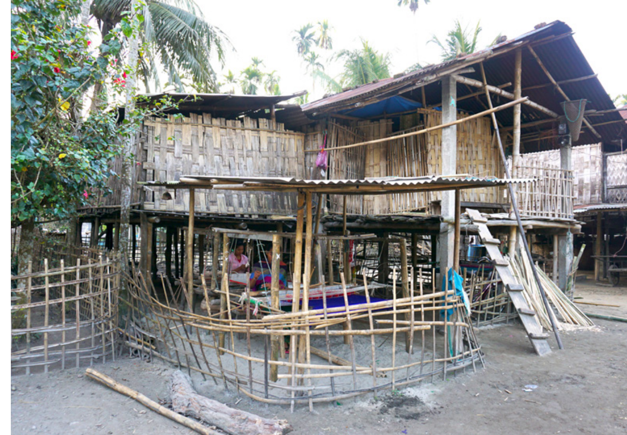
'Chaang ghars' Bamboo constructed houses raised on stilts. Weaving is practiced in the still-level. Photo credit: Shivali Gaikwad
