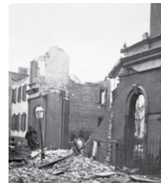
Remnants of the Brooklyn Theatre facing Johnson Street after the fire of December 5, 1876. The wood interior structure has entirely burned away, leaving only pieces of the exterior masonry walls. Photo by Waller & Schrader, Photographers, published as a stereograph.
