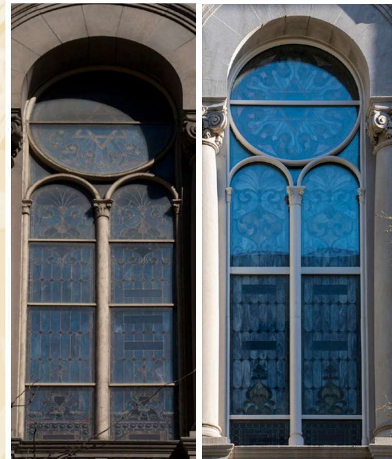
Left: South facade window prior to the fire. Right: South windows from the interior after restoration with the blast mitigation glazing in place. Photos courtesy of author.
