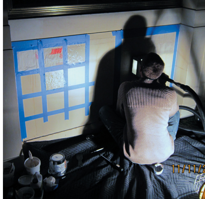
Blast cleaning at Waldorf-Astoria Lobby. Photo Credit: Ken Follett Left: Aggregate blasting at The Elms, Newport, RI. Photo Credit: Ken Follett
