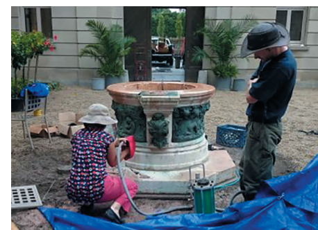
Blast cleaning at Waldorf-Astoria Lobby. Photo Credit: Ken Follett Left: Aggregate blasting at The Elms, Newport, RI. Photo Credit: Ken Follett
