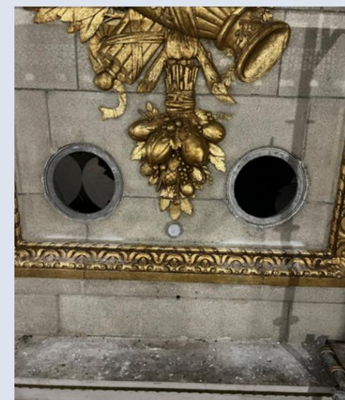
North light holes in the wall that need patching with Sphinxstone. Photo Credit: John Canning & Co., Ltd.
