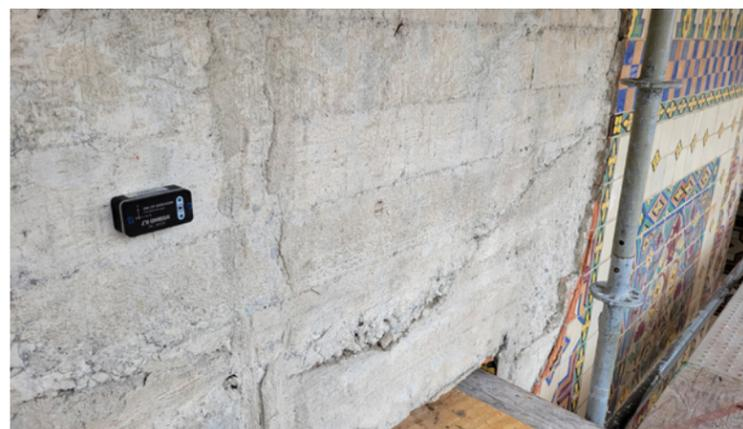
Detail of vibration monitor installed at location of tile failure, 2022. Photo Credit: McGinnis Chen Associates, Inc.
